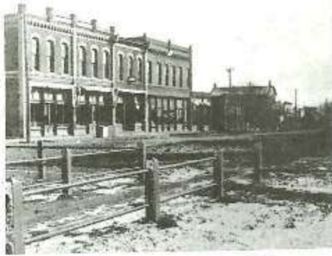
South view of Railroad after 1908.
