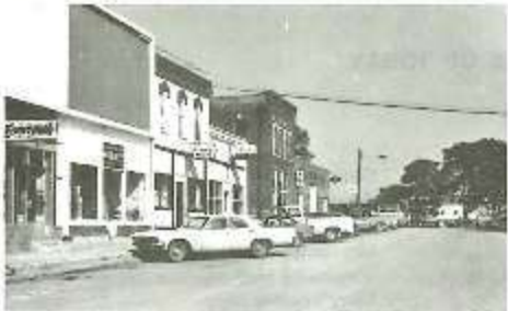
Econ—O—Wash—American Legion (Centennial headquarters)-Gerety Heating-Air Cond.-Potts Impl.
