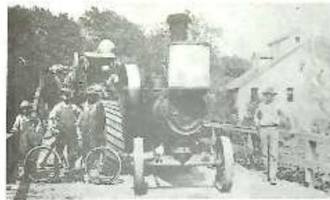
Mooney steam engine on Arrington bridge and mill in background.
