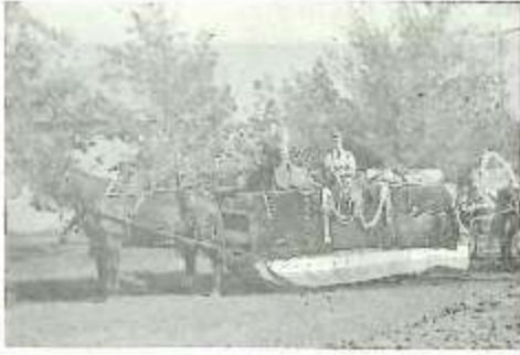
F. C. Baur Harness Shop Float early 1900.
