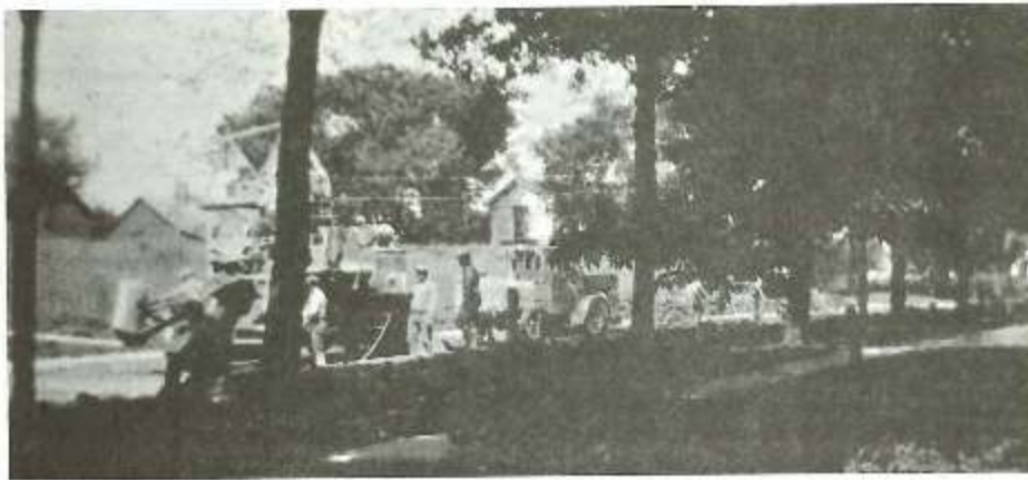
Paving of Locust Street in front of the now Fred Schuler and Ira Bond residences, in 1925.
